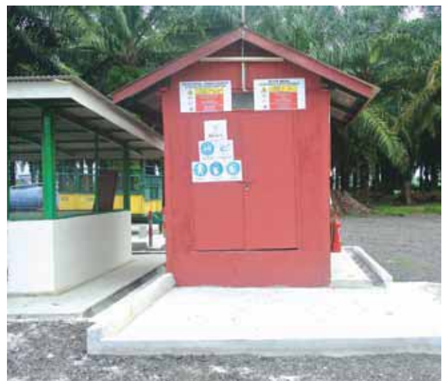
New buildings for the separate storage of chemicals and other materials
